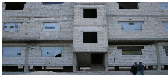
Rehabilitation of 360 shelters of the Syrian Rsfugees in Al Gizlanieh:
