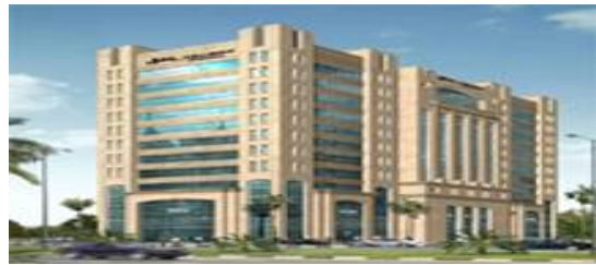
SyriaTel - Data Center
