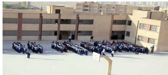
Rehabilitation Works of Eight Schools
